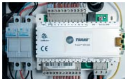
Typical ZN523 factory mounting (metal cover removed)
